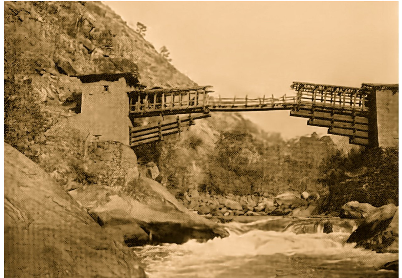
Cantilever Bridge over the Kulong Chu, Eastern Bhutan.
